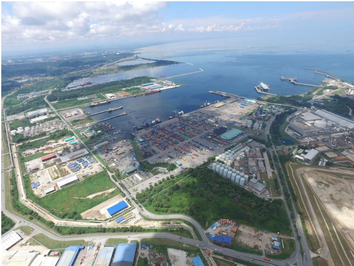
Figure 4 Aerial view of current Bintulu port
